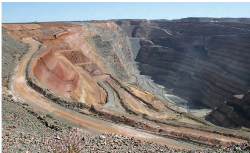
Overall view of the mine. The white or orange coloured areas indicate quartz containing gold, while the grey indicates dolomite, but also with some gold, and the black stripes are carbon (burnt and compressed organic matter). There is currently no technology to extract gold from rock chemically, so the process is all down to grinding and separation on the basis of density.
